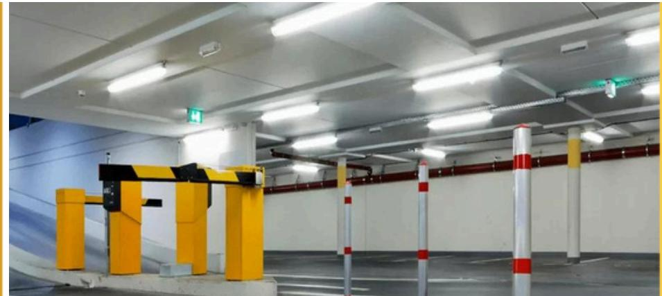
LUMINÁRIA HERMETICA BLINDADA PARA 2 LÂMPADAS TUBULATRES T5 OU T8. BORRACHA EXPANDIDA PARA VEDAÇÃO, CORPO EXTRUSADO EM PVC CINZA ANTI-CHAMAS, TAMPA LATERAL INJETADA EM NYLON, PRENSA CABO EM NYLON, PLUG ALIMENTADOR INJETADO, DIFUSOR EXTRUSADO EM PVC CRISTAL ANTI-CHAMAS, PLACA DEMONTAGEM EM PVC BRANCA, SUPORTE INJETADO EM NYLON
